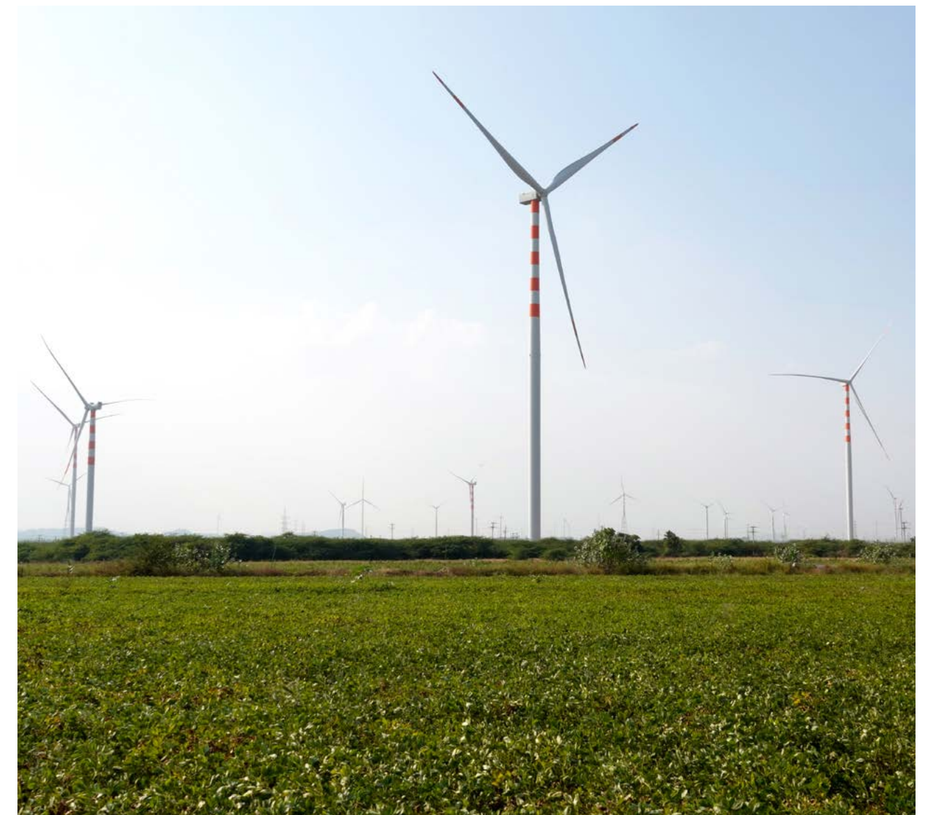
Figure 5: Wind Turbines at Morjar Site
